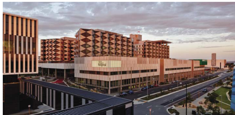
Fiona Stanley Hospital, Murdoch Western Australia
